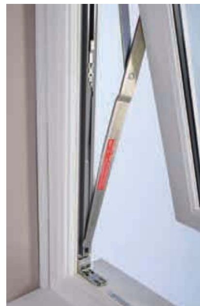
Top Swing restrictor second position
