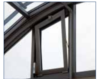
Fanlight opener system with electric linear drive
